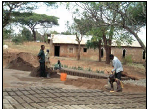
Preparing The Concrete Blocks
